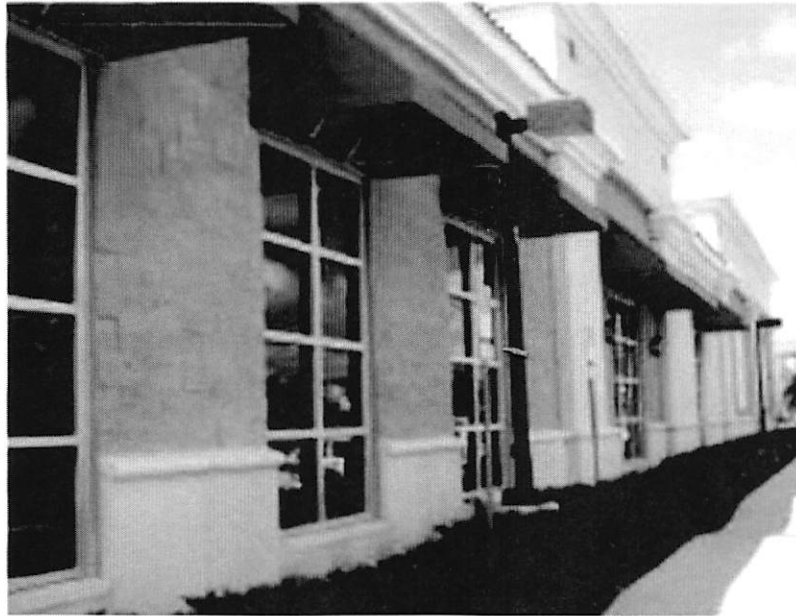
1 2 Figure 4 - Pedestrian-Scale facade with fenestration 3 covering a minimum of 40% and maximum of 80% 4 of occupants' linear frontage
